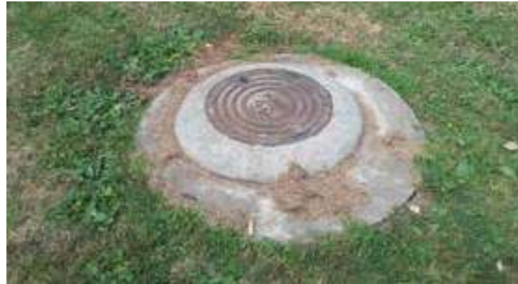
Exposed manhole on grassed area
