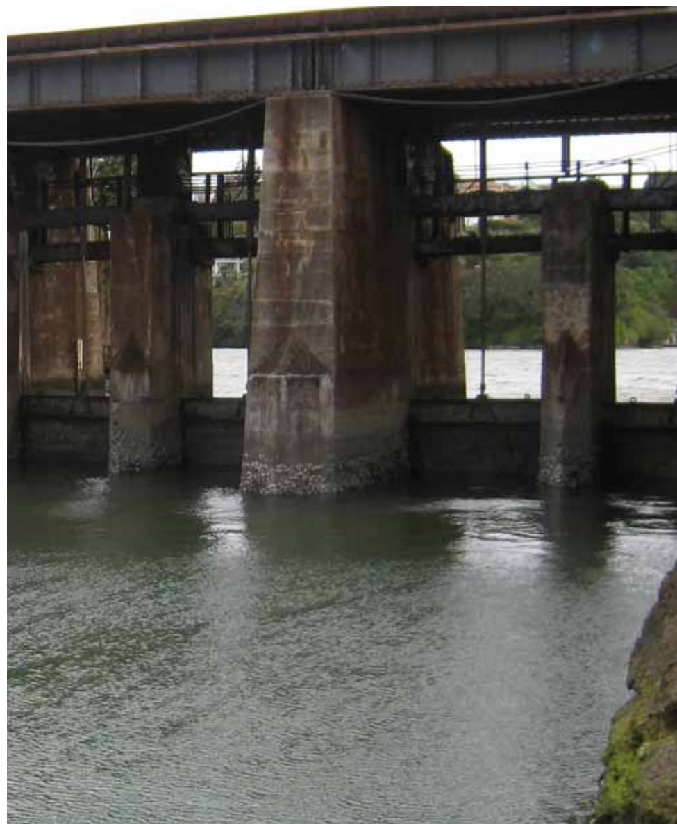
Sluice gates: circa 2008
