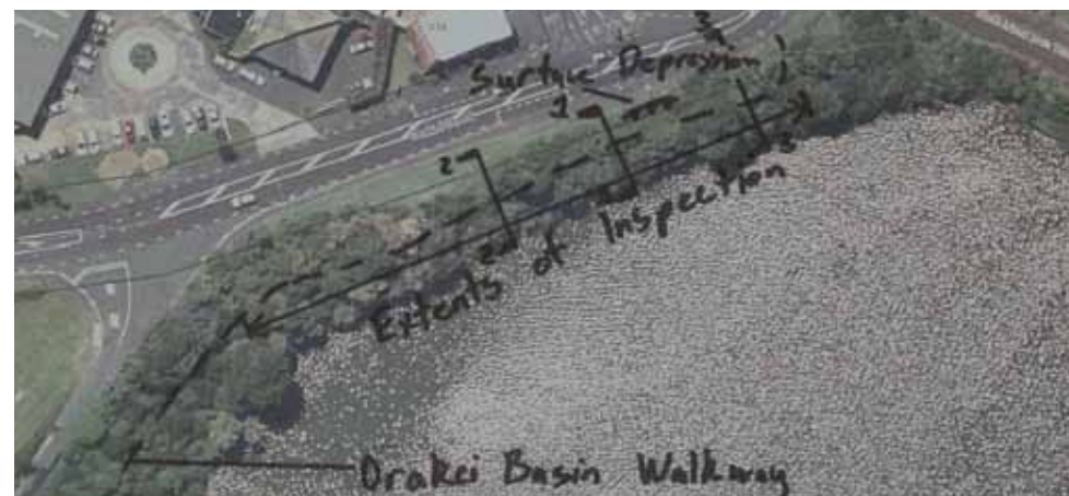
Source: Tonkin & Taylor 1 August 2008 Orakei Basin Visual Assessment of Slope Stability
