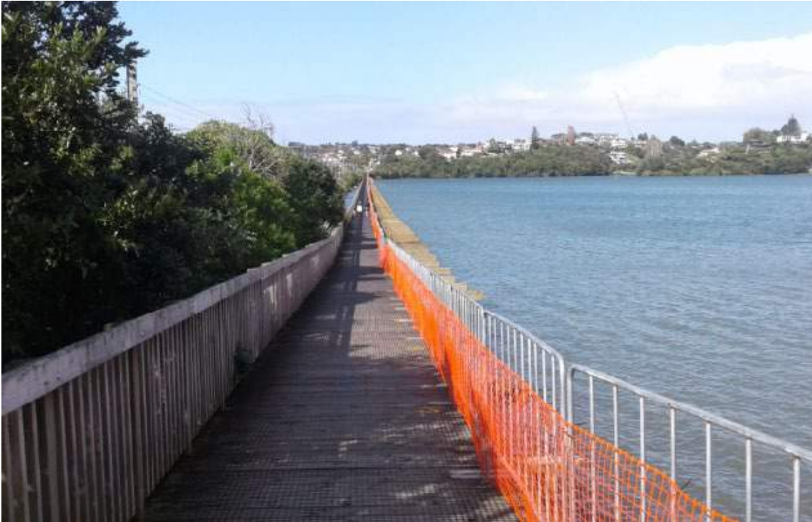
Figure 17: Upgrade works on the railway embankment boardwalk across Ōrākei Basin
