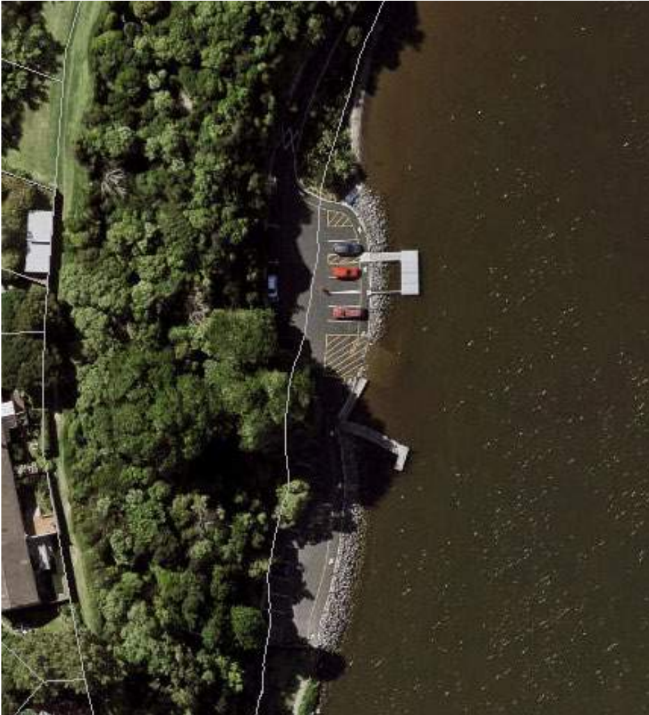
Figure 34: Examples of existing water access points
