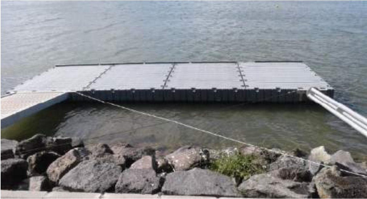
Figure 18: Pontoon structure accessed from the main car park
