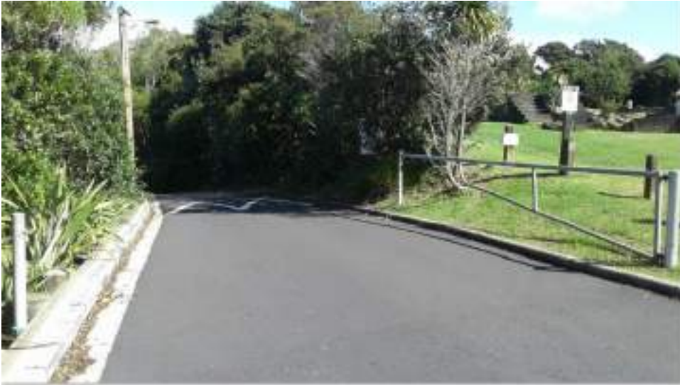
Figure 35: The upgraded access road and entrance from Ōrākei Road
