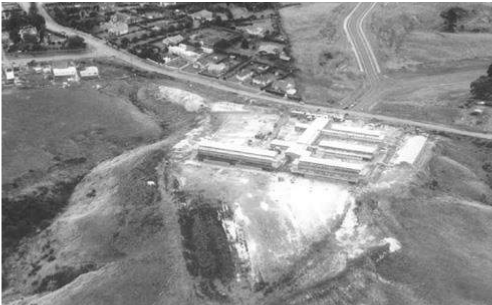
Figure 2 Selwyn College construction (1956)
