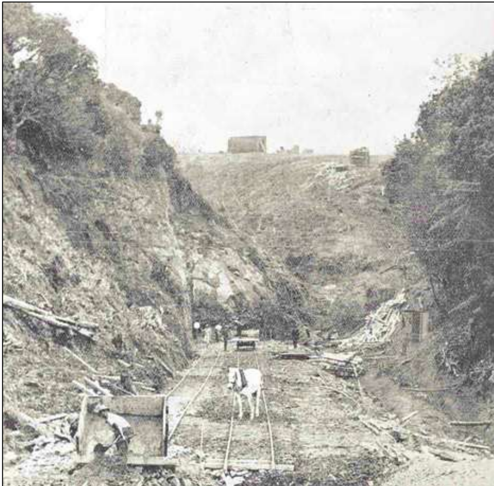
Purewa Tunnel Construction in 1925 New Zealand Herald Glass Plate Collection; Auckland Libraries Heritage Collections AWNS-19250507-54-4
