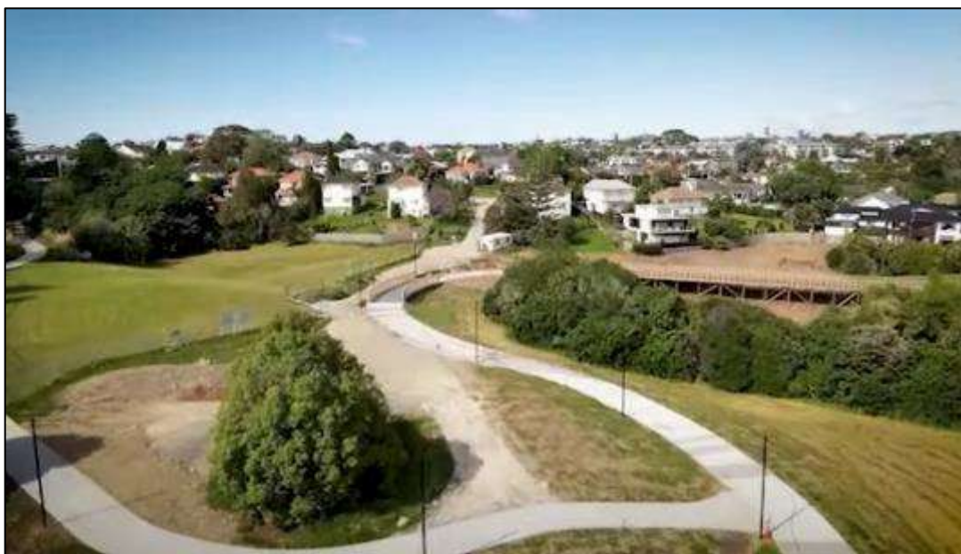
December 2021 view of shared pathway through Tahapa East Reserve from Waka Kotahi Project Update Video 21-12-2021
